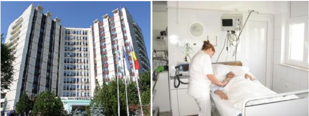
Fig. 1 – Photographs of the studied hospital: a) North and East aisle; b) Interior of a renovated hospital ward.
