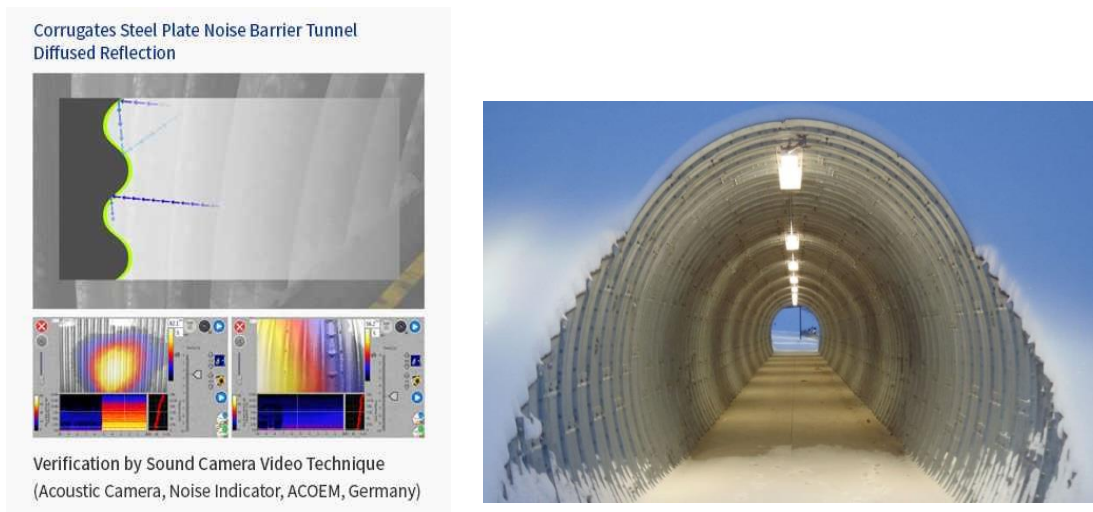
Fig. 9 - Applying of corrugations in auto-tunnels and measurements done with sound camera [5]
