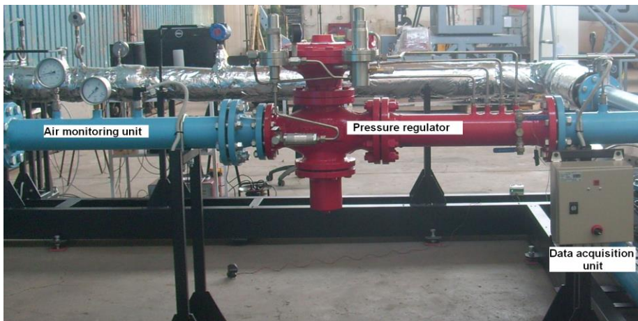
Figure 6. Air conditioning unit – photo of air monitoring, pressure regulator and data acquisition unit
